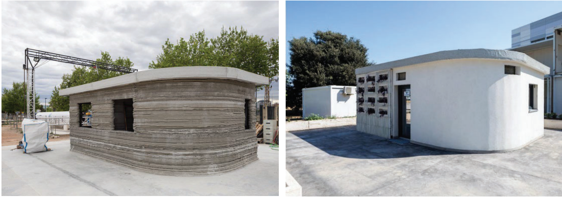
Figure 3. First 3D printed house in Spain
